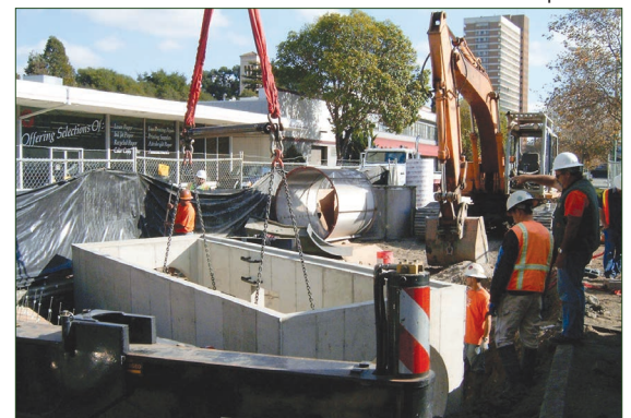
Installation of a trash separator
