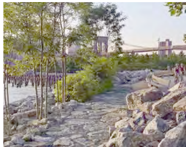
FITTED STONE PAVING AND STACKED RIPRAP
